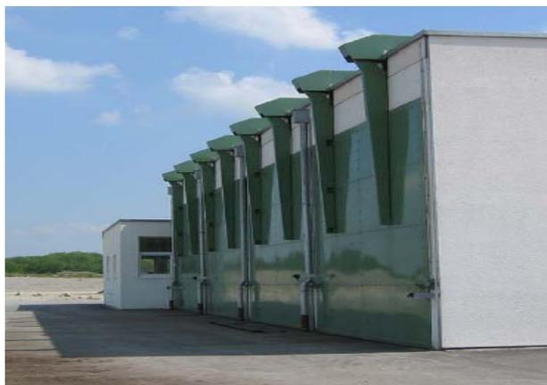
*Closed tunnel reactors for dry fermentation.*
